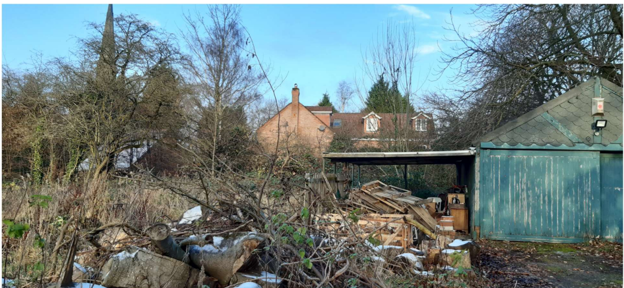
Photo 8: View of the site and the existing garage
